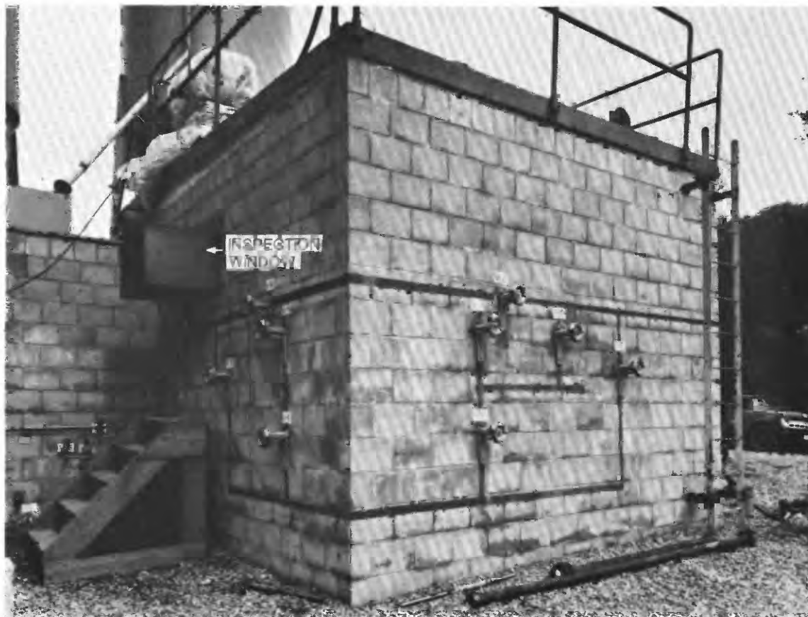
FIGURE 44. – Photograph showing cell enclosing the wellhead of the waste-injection well, Oak Ridge National Laboratory, Tenn. (Courtesy of Oak Ridge National Laboratory.)
