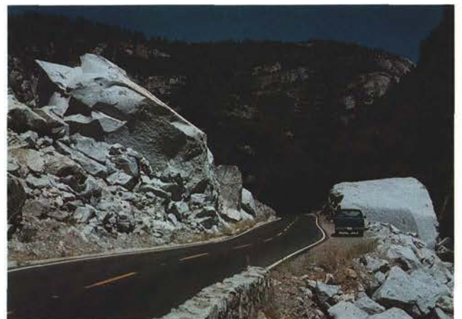
ROCKFALL of blocks the size of small houses temporarily closed the El Portal Road east of Arch Rock Entrance Station in 1982 until a way could be blasted through the debris. (Fig. 49)
