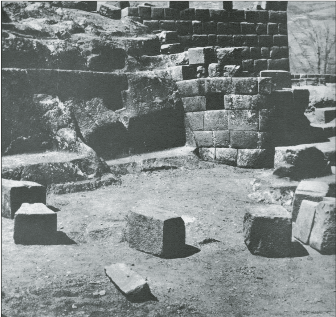
Figure 8. Pisac ruins at Cusco which were constructed using building blocks that were finished only on the exterior surface (see Chapter 1). (Photograph by Prof. F. Corante, 1970.)
