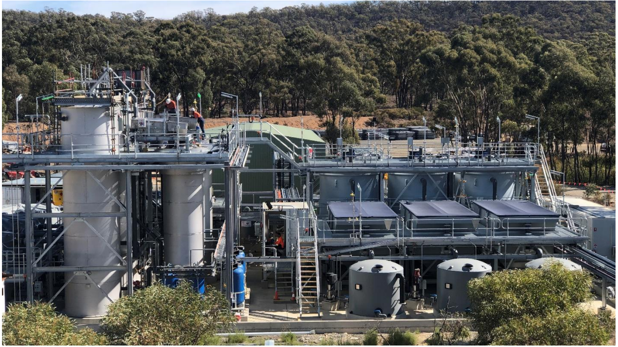
Figure 6. Photo of the Completed Plant
