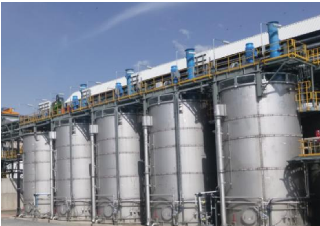
Figure 5 Albion Process™ Oxidative Leaching Train
