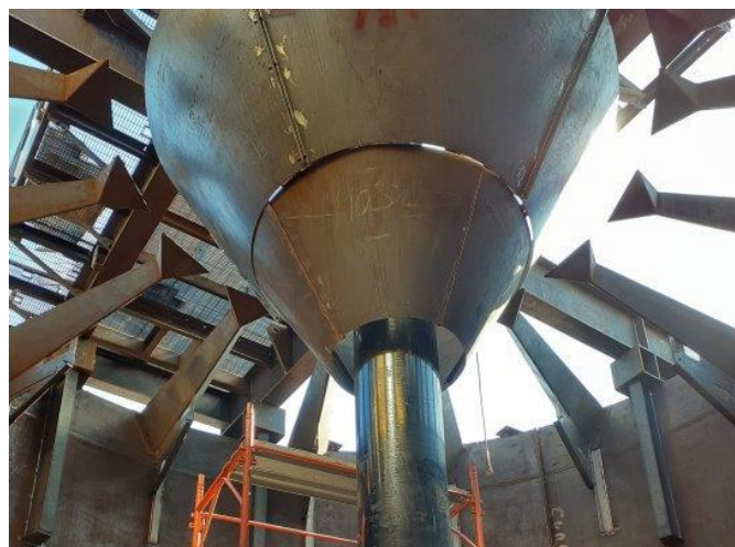
Figure 6: Central Cone Crowder surrounded by High Efficiency Radial Launderers.
