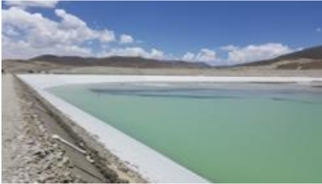
Figure 6. Las Bambas. Geocomposite installation at Stage 2 (height 118 m).
