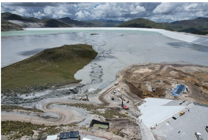
Figure 8. Las Bambas. Geocomposite installation at Stage 4 (height 173 m), current situation.
