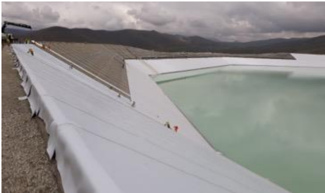
Figure 7. Las Bambas. Geocomposite installation at Stage 3 (height 148 m).
