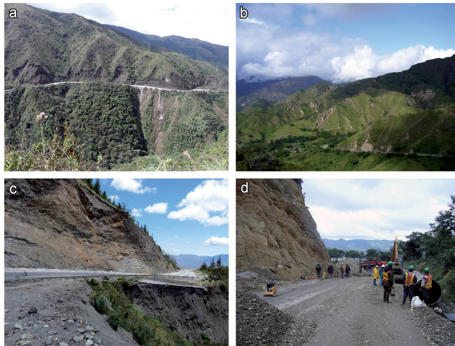
Figure 2. Landslides occurring along the investigated highways. (a) Typical landslides of the wet metamorphic part of the study area in the east. (b) Typical landslides of the semi-arid, conglomeratic part of the study area in the west. (c) Highway destroyed by landsliding. (d) A highway is cleared from a recent landslide occurrence.
