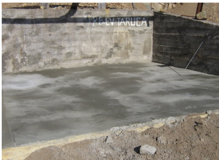
Figure 47 -Reclamation of Ventilation Raise
