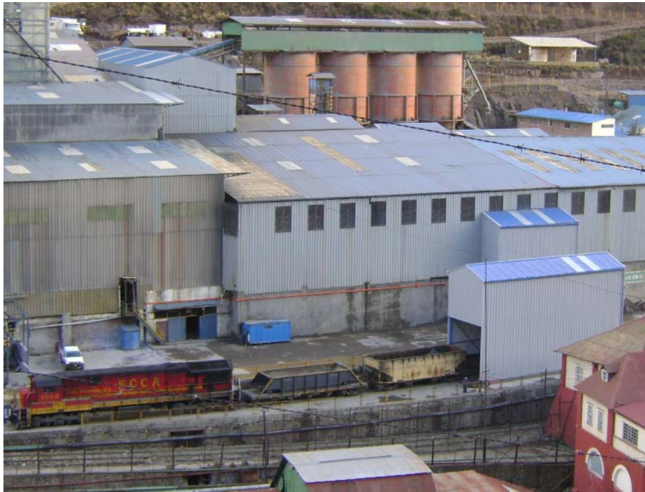
Figure 45 -Rail Load-Out Facility
