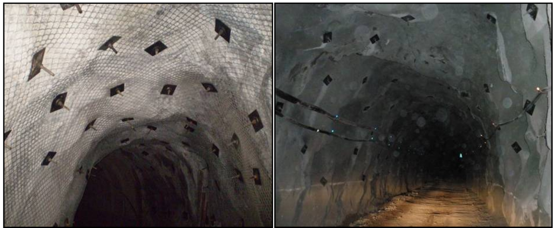
Figure 42 -Typical Ground Support (mesh + bolts, shotcrete + bolts)
