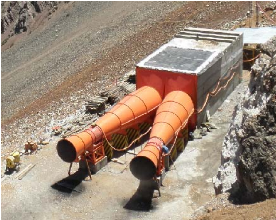
Figure 36 -Troncal #4 Fan Installation (4,800 masl)
