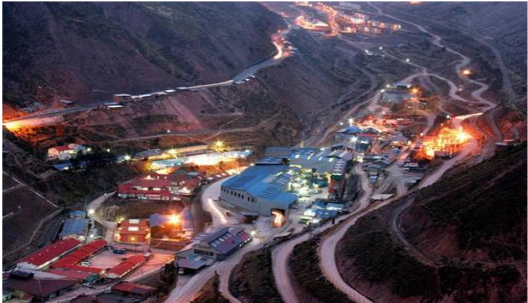
Figure 25 -Yauliyacu Process Plant and Administration Buildings
