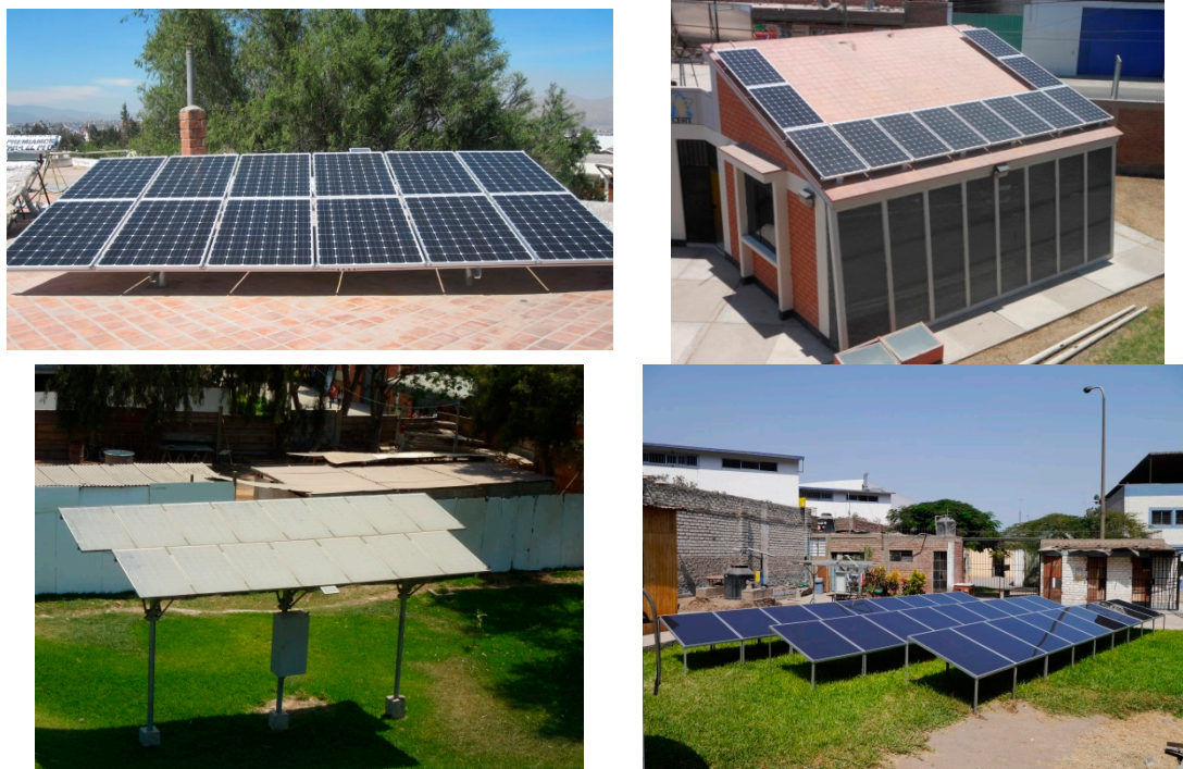
Figure 1. Photographs of the PV systems under investigation. (Top left) PVGCS #1 in Arequipa (sc-Si, installation on flat roof); (top right) PVGCS #2 in Tacna (sc-Si, building integrated installation); (bottom left) PVGCS #2 in Lima (mc-Si, on-ground installation); (bottom right) PVGCS #4 in Lima (a-Si/ \mu -Si, on-ground installation).
