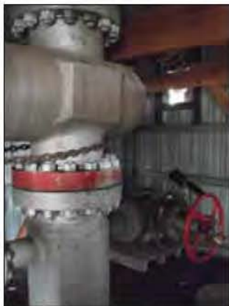
Protective housing surrounds a geothermal well head. PHOTO BY F. ECHAVARRIA.
