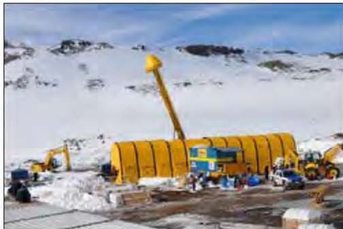
Drilling the slim hole MP 03 in the snow at the Maule Geothermal Project in 2010, 2,400 m above sea level. The seasonal snowfall exceeded 5 m. PHOTO COURTESY OF ALTERRA POWER
