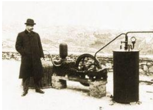
Figure 3: The engine used at Larderello in 1904 in the first experiment in generating electric energy from geothermal steam, along with its inventor, Prince Piero Ginori Conti.
