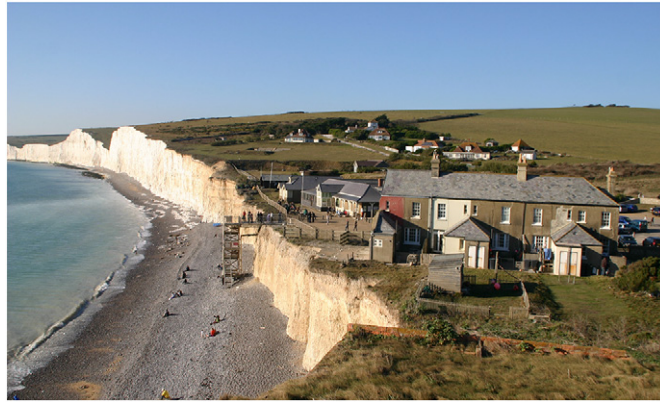
Fig. 8. The eroding coastal cliffs at Birling Gap, southern England.
