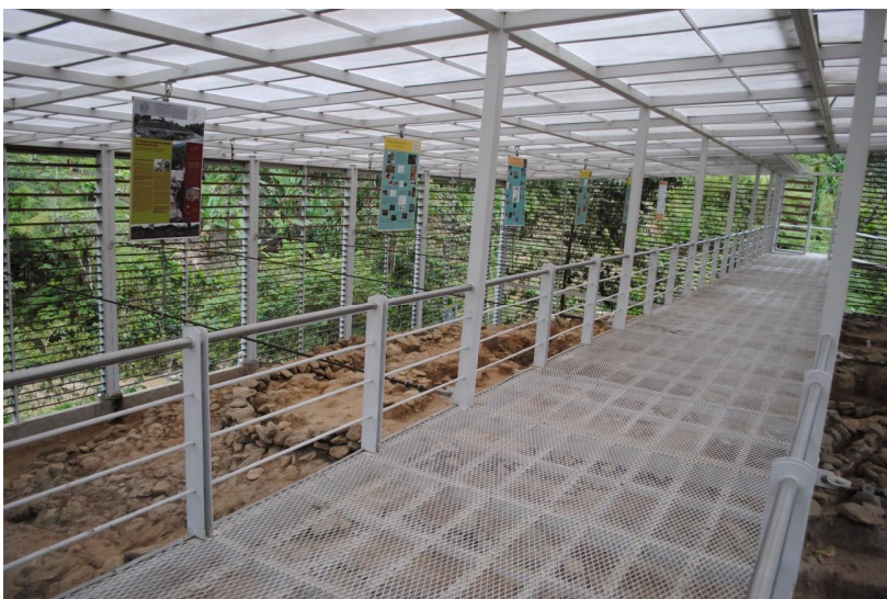
Figure 4 Hanging bridge platform and information panels.
