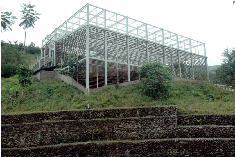
Figure 3 Interpretative center structure protects ancient architecture.
