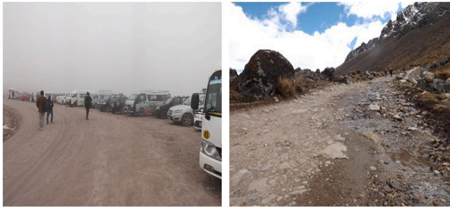
Fig. 4. Severe deterioration of Trail 1 due to excessive vehicular traffic.
