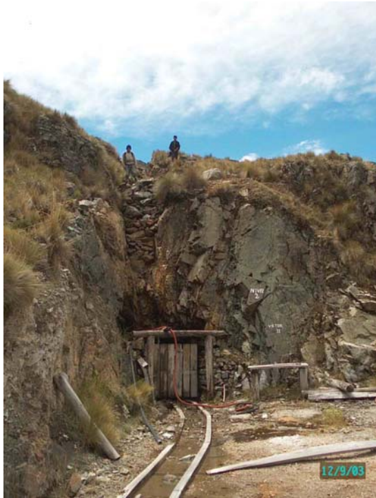
Photo 2: Victor I Adit. Notice wooden rails and strength of structure
