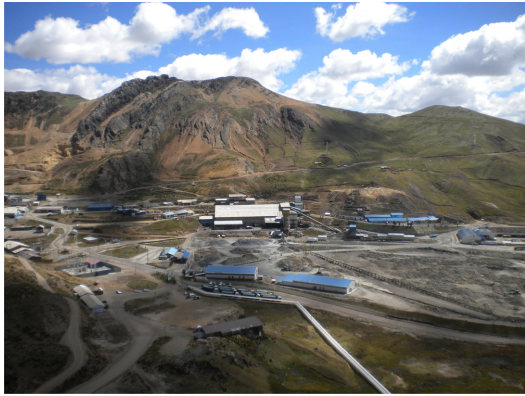
Fig. 11. Photograph of Huaron mine.
