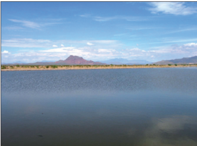
Figure 2. Recharge basin of the Granite Reef Underground Storage Project. This basin has a surface area of 25 hectares and an infiltration rate of one meter per day
