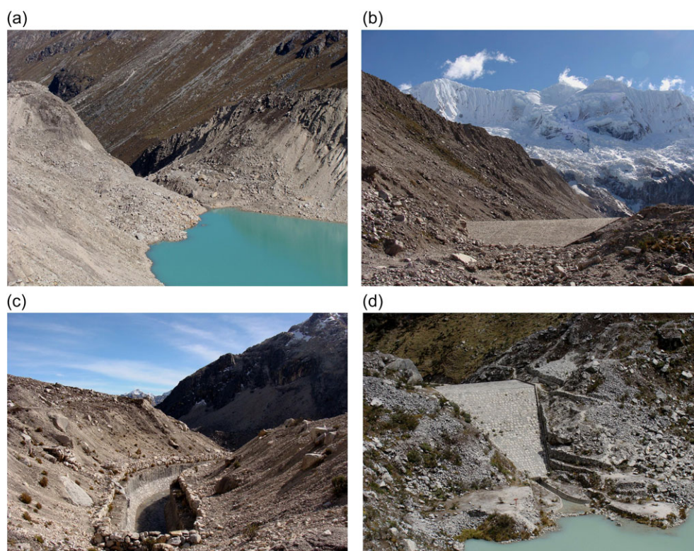
Figure 2 Example of open cuts and artificial dams. (a) A failed moraine dam of Lake Milluacocha equipped in 2000 with an open cut; (b) a separate artificial dam increasing the dam freeboard of Lake Palcacocha in the naturally lowered part of the dam crest (not the lake outflow); (c) a downstream view of the open cut of Lake Ishinca from an artificial dam providing a freeboard of 5 m; and part (d) an artificial dam providing a freeboard of 12 m and an inlet to the open cut draining Lake Llaca.
