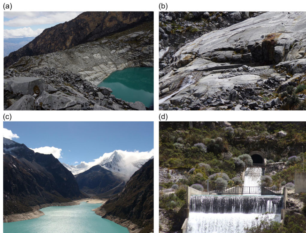
Figure 3 Examples of lakes equipped with tunnels. (a) A bedrock dam of Lake No. 513 partly covered by moraine material, and the debris-free bedrock indicates the original water level before being lowered 20 m; (b) the outlet of a tunnel dug through the bedrock dam of Lake No. 513; (c) an overview of Lake Parón from the Jatunraju glacier damming the lake (note the light belt around the lake indicating a decrease in the water level of about 40 m); and (d) the outlet of the tunnel below Lake Parón.
