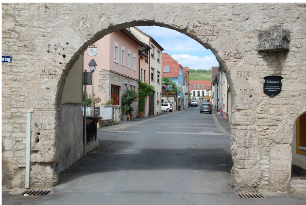
Fig. 5 Flood marks in the town of Eibelstadt, river Main, Germany (photo by P. Migoñ)
