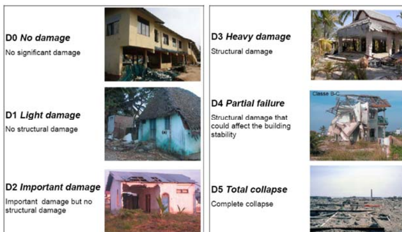
Figure 23: Examples of damage to buildings associated with the damage matrix proposed in Table 6. Figures are from the 2004 Indian Ocean tsunami (sources: Leone et al. 2010, Peiris 2006 and Garcin et al. 2007)
