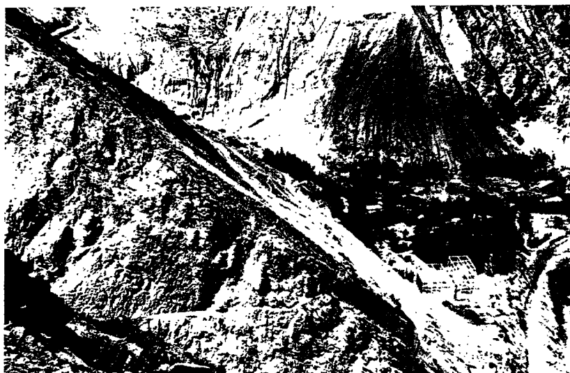
Fig. 4 - Parallel oriented pattern of granodiorite, along which cleavage occurs under seismic loading, thus menacing the transformer platform of the hydro-electric plant at Huallanca.
