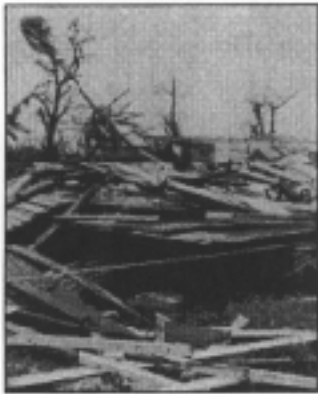
Hurricane damage in Nicaragua, 1988. UNDRO NEWS, May/June 1989.
