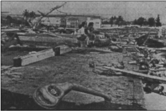
These broken utility pole and bent parking meters were the result of tsunami waves which occurred May 22, 1960 at Hilo, Hawaii.
