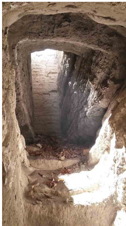
FIG. 5A. Typical shaft well ( lumbrera ) in the Pica area.
